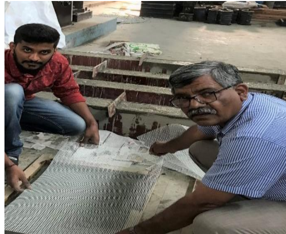
Fig 1 (a): Preparation of reinforcement
